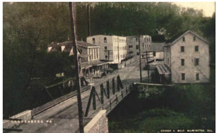
A view of the Landenberg Bridge early in the 20th century. The Landenberg Hotel, the Store, and the Lund Woolen Mill can be seen behind the bridge. On the right is a tenant house for mill workers.
