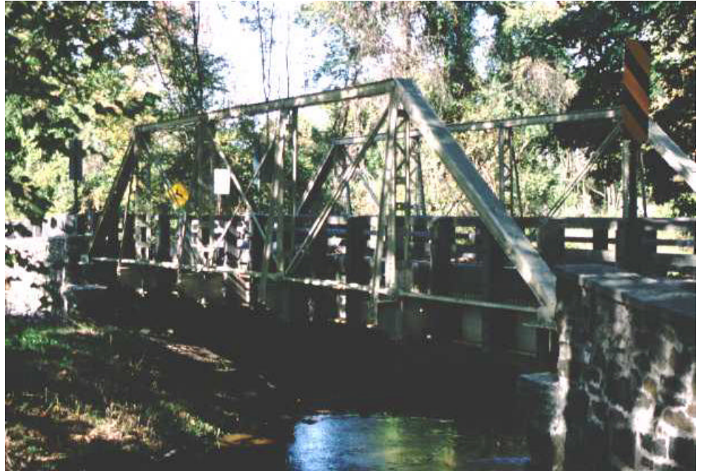
The excellent restoration of the Wollaston Rd. Bridge north of Kennett Square done by Chester County in 1992 is seen as an example of what should be done for the Landenberg
